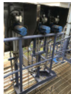
FIG 3 Three Yokogawa transmitters installation.
